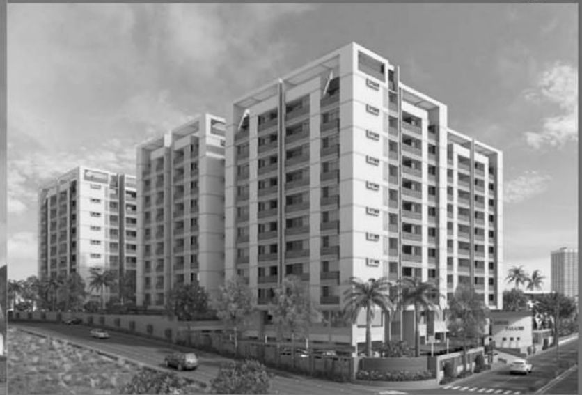
100 FT. ROAD, SOBHAGPURA
