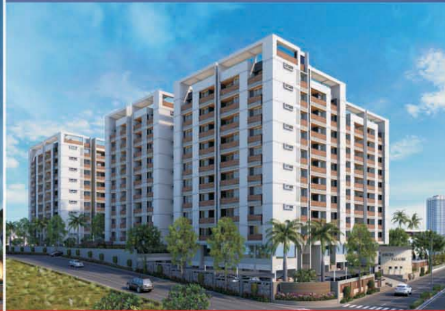
100 FT. ROAD, SOBHAGPURA
